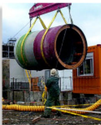
A 72-inch diameter intermediate jacking station section being lowered into the jacking pit.
