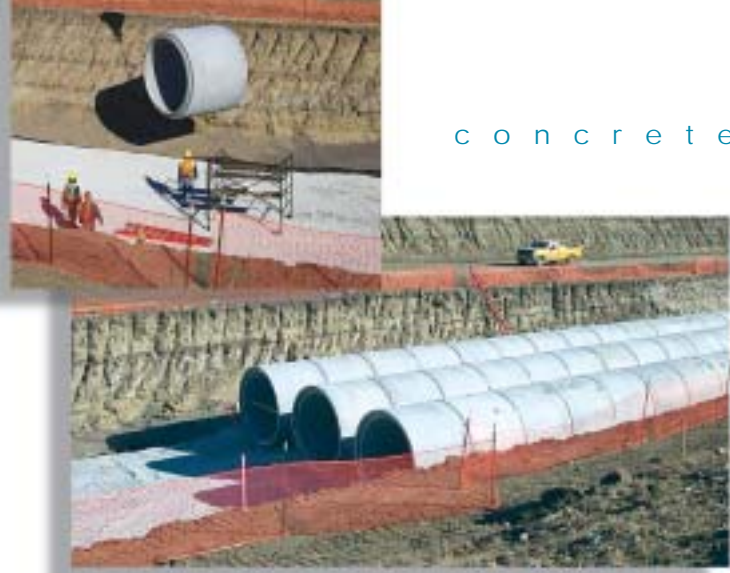
A portion of the storm and sanitary sewer infrastructure for Omaha's waterfront project consists of a triple line of 108-inch diameter RCP.
