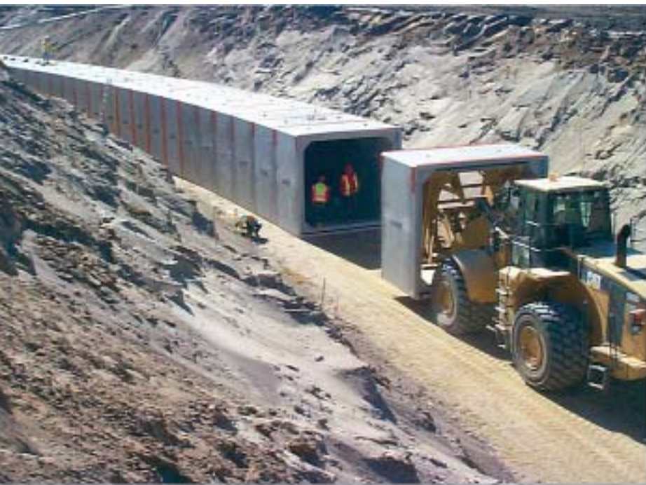
781 dry-cast concrete box sections were provided for the 4,777-foot long storm sewer in Phase I of the airport drainage system expansion.
