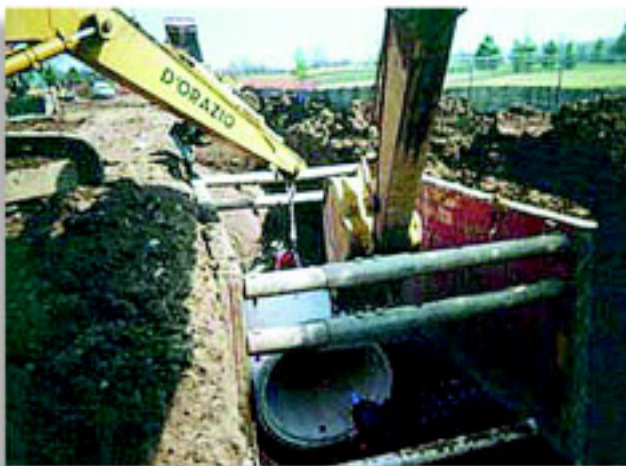
A fast-paced schedule and safety considerations required the use of trench boxes for much of the 15.5 kilometers of RCP installed along the Highway 25 right-of-way.
