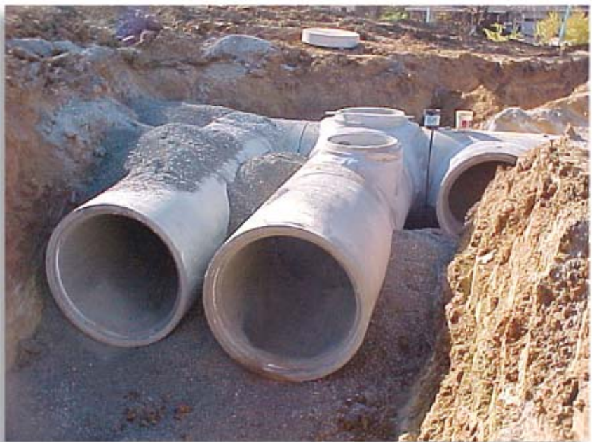
Installation of the 72-foot runs of 66-inch diameter RCP went smoothly and provided the owners with the ability to add a parking surface above the structure.
