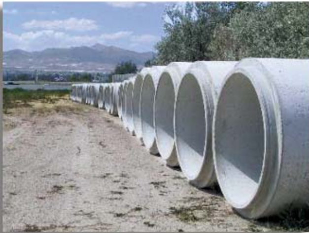
60-inch and 48-inch diameter RCP was staged for installation along Interstate 15 in Sandy City. Utah's Oquirrh Mountains provided a scenic backdrop for crews.
