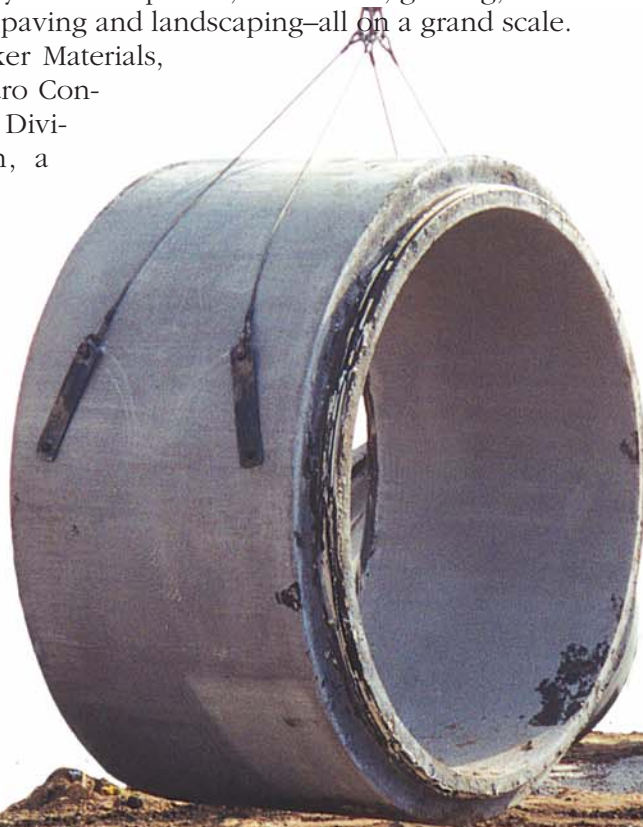
A 7-foot section of 144-inch diameter 1350 D RCP (with gasket on and spigot/gasket soaped with lubricant) is lowered into the trench for installation.
