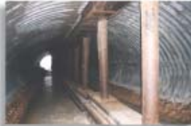
Steel struts and wood beams were used to support the excessively deflected SPCSP...
