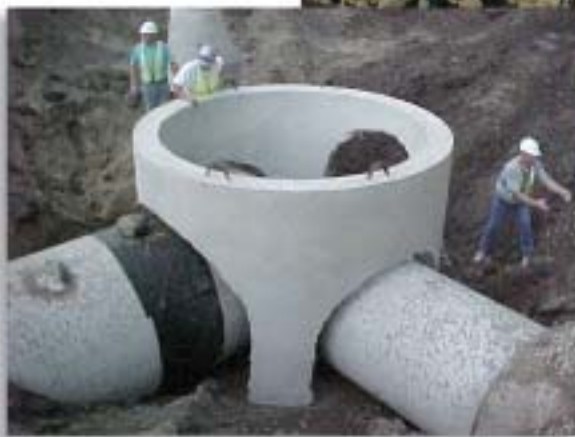
Several multi-inlet precast structures were fabricated by North Dakota Concrete Products Company for the South Broadway project.
