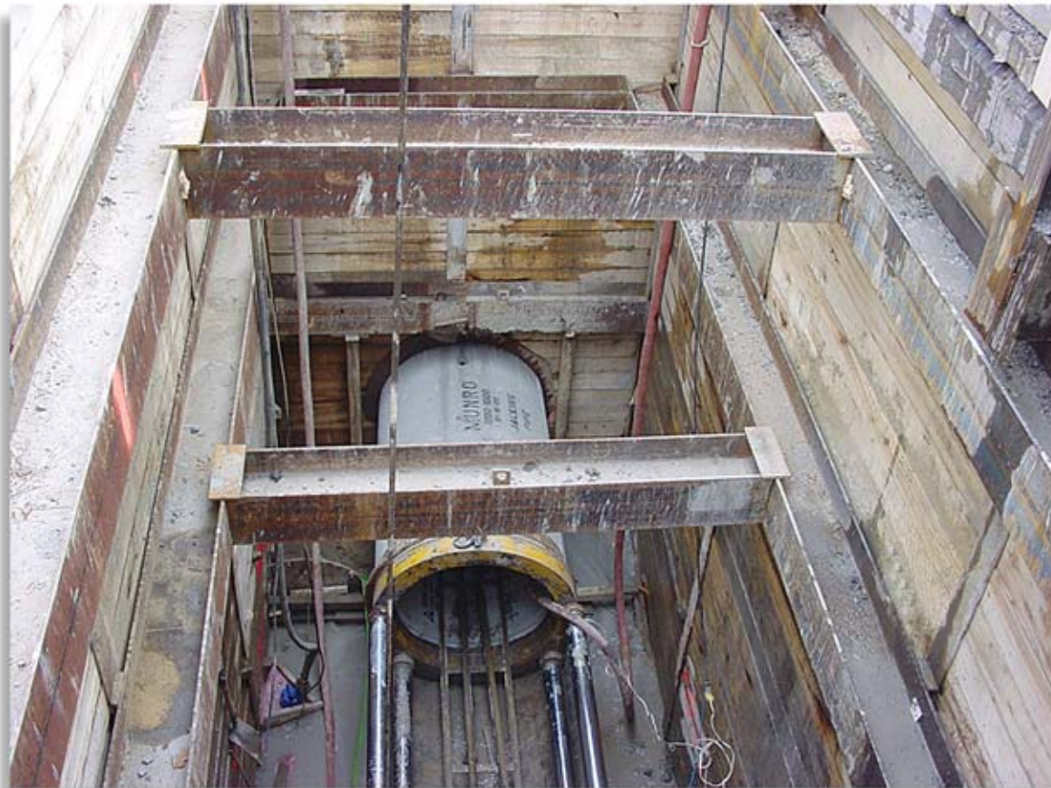
Two different jacking contractors, working from two locations, enabled Toronto's Works and Emergency Technical Services Department to complete the 1200 mm, 100 D (48-inch diameter Class IV) jacking project in only 90 days.
