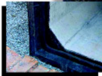
Closed-cell neoprene joint sealant was applied to the bell of each box section prior to shipment to the job site.
