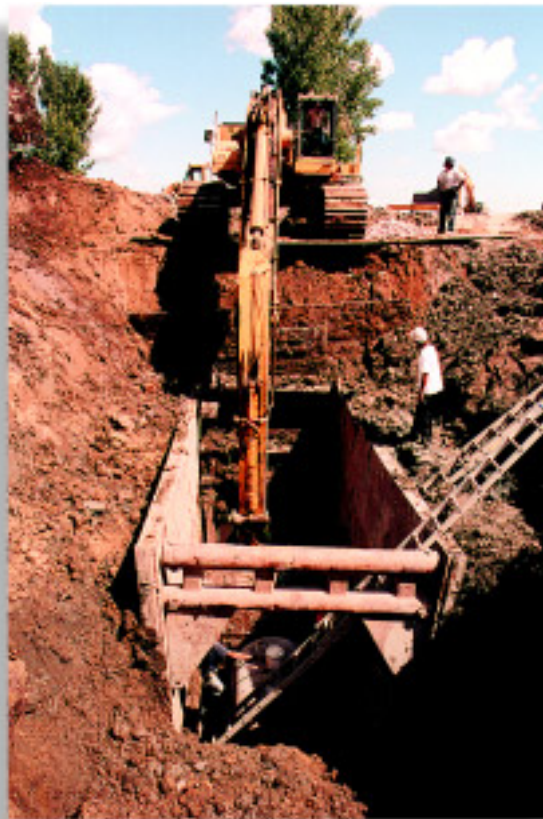
6,900 meters (22,638 feet) of precast reinforced concrete pipe was used for the Matte Collector System. The line was designed to accommodate flows from sub-basins.
